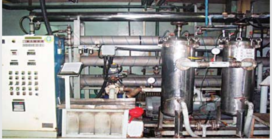
Reverse Osmosis System
