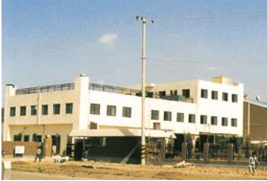
The construction of Ansan factory (formerly KISCO) was completed (September 1984)
